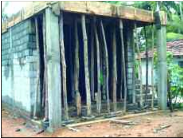
Credit union being re-built
